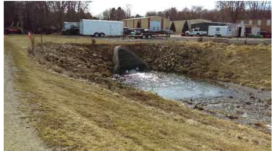
4) Adjacent culvert near southwest corner
