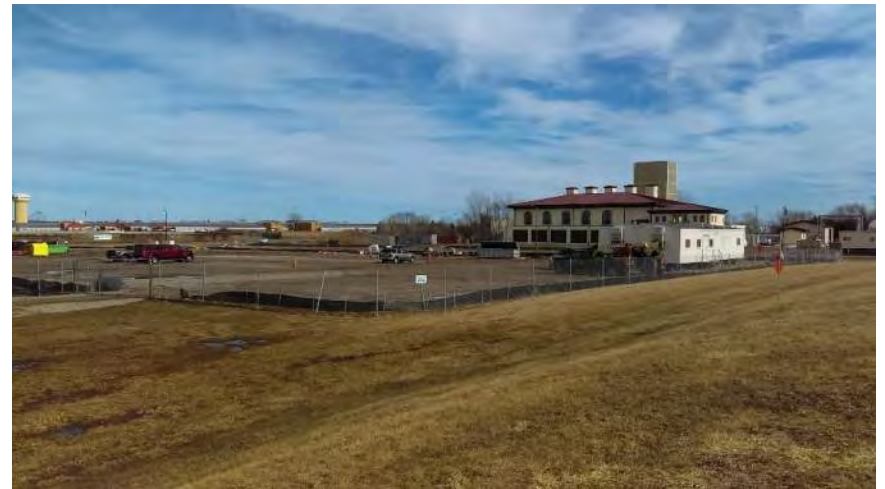
12) Contractor parking and trailer on southwest portion of Subject Property
