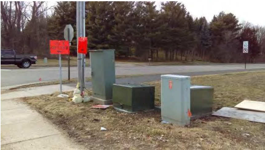
11) Southwest corner of Subject Property
