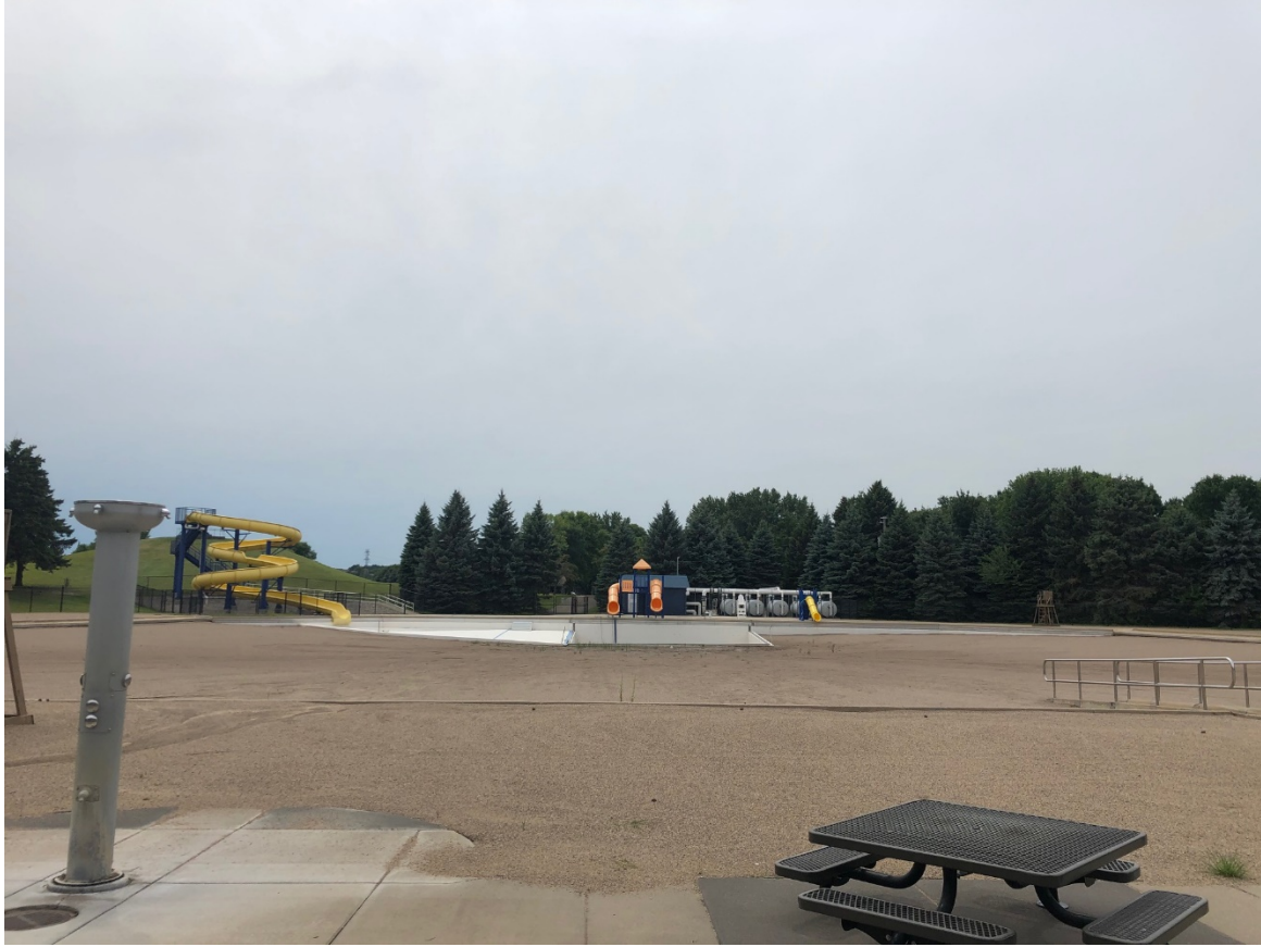
Interior of SandVenture Pool Decking and Zero Entry Pool
