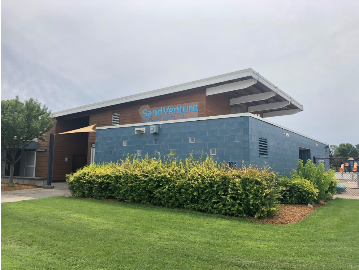
Exterior of SandVenture Pool Building
