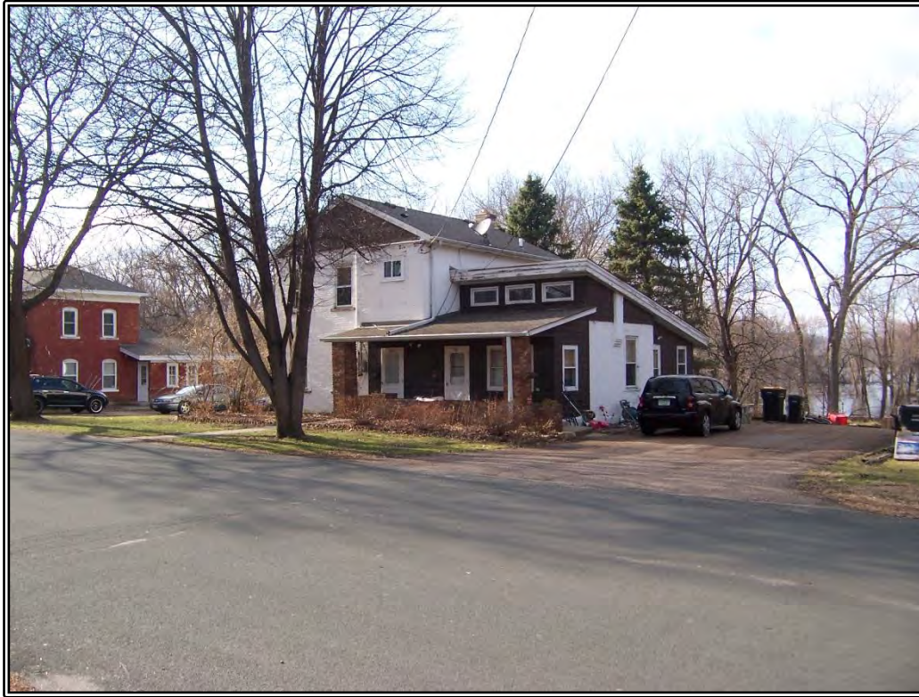
View to NW at 731 Bluff Ave. E.
