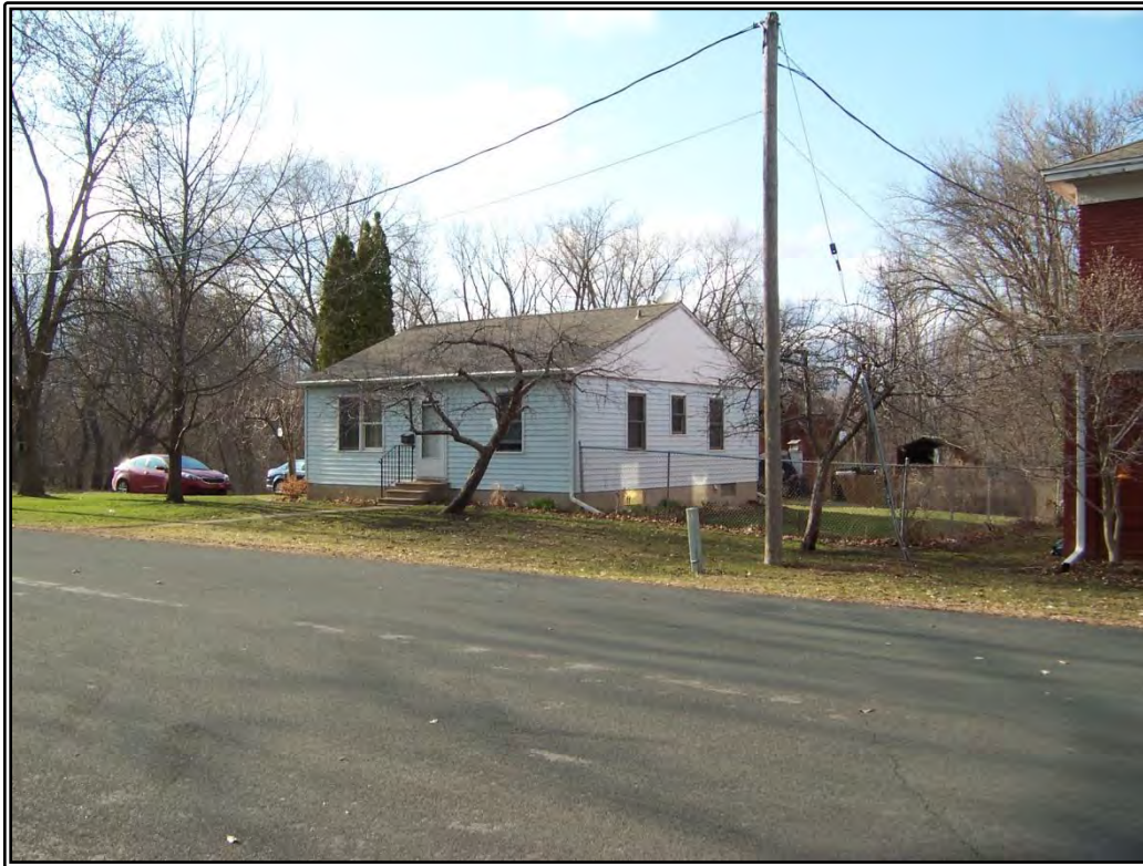
View to NW at 711 Bluff Ave. E.
