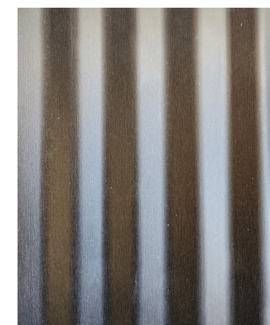
CORROGATED METAL SIDING (IRON ORE)
